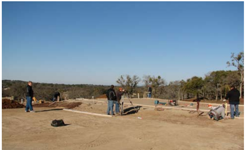
Gary Beam begins Clergy Residence Construction
